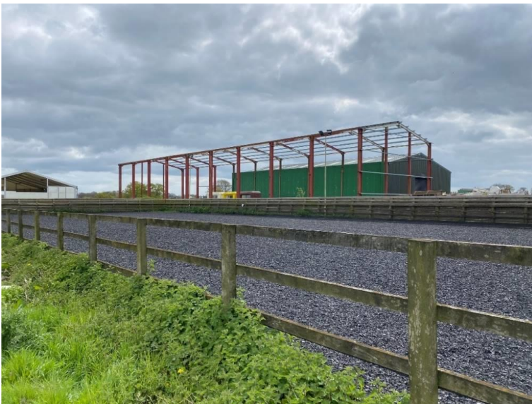
Photo 1: The Manege, Temp Building 1, steel frame of Building 7, and Building 8
